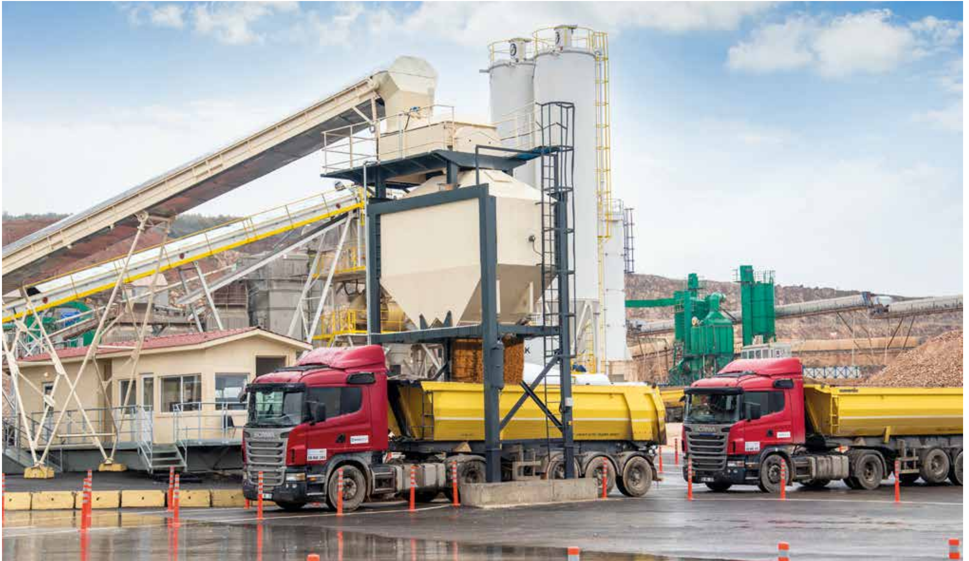
Cold Mix (Mechanical Stabilization) Asphalt Plant
