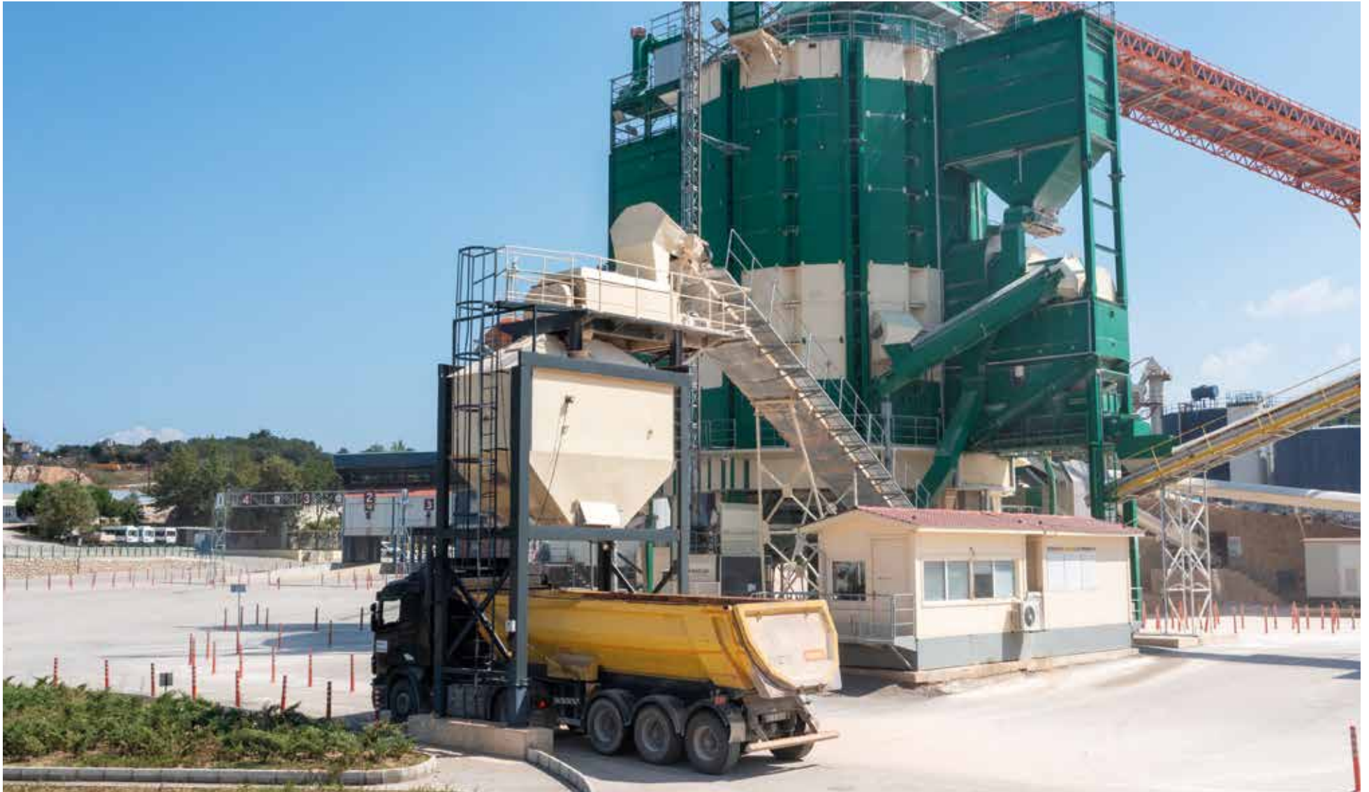
Cold Mix (Mechanical Stabilization) Asphalt Plant
